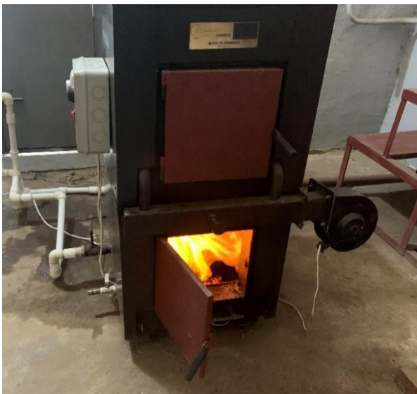
Figure 10: Pyrogenic boiler (Barva center)
